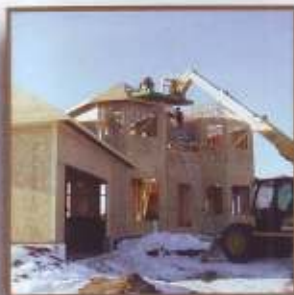
Day 5 - Sheathing roof
