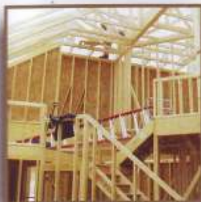
Day 4 - Putting up roof trusses
