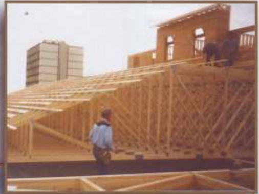
Construction on the Ramada
