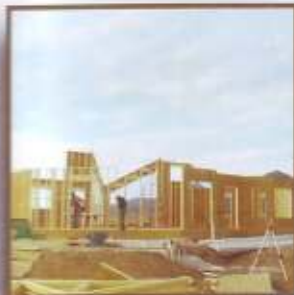
Day 3 - Building exterior walls
