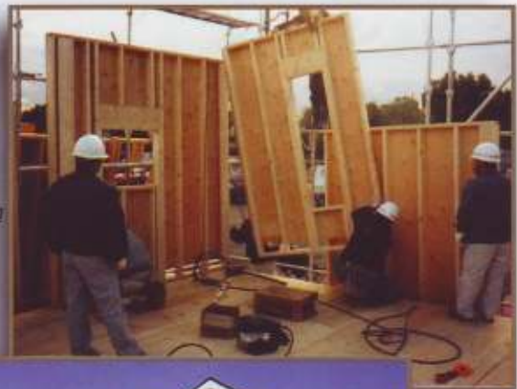
Assembling Nelson panelized walls in Japan
