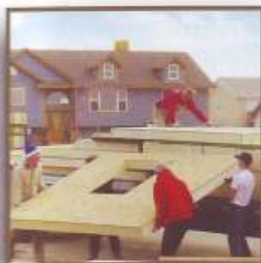
Day 1 - Unloading wall panels
