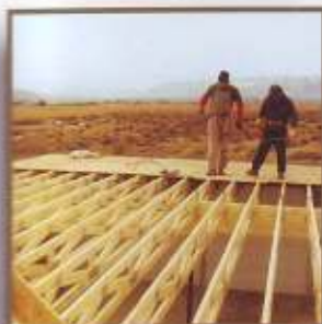
Day 2 - Sheathing floor
